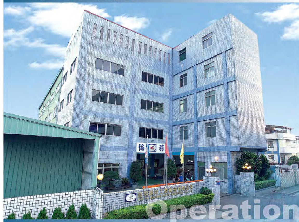
協羽高雄廠一廠 Kaohsiung Plant I
